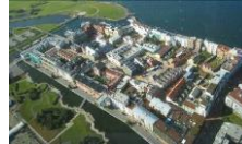
Western harbour/Bo 01 Malmö
