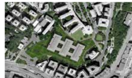
Figure 3: Aerial view of Galliera Hospital Site showing new hospital buildings in the centre of the site
