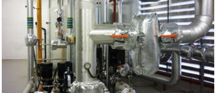
District heating in Southampton
