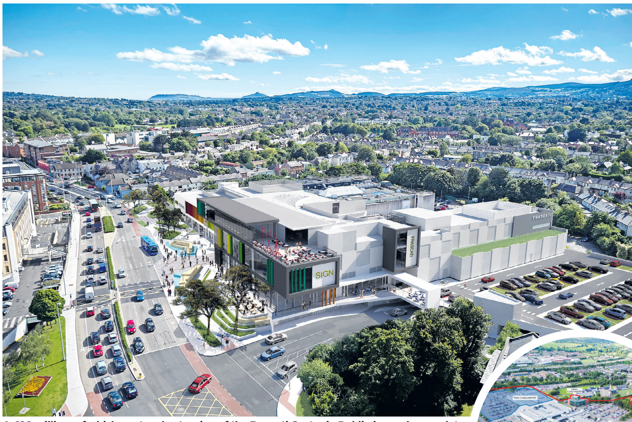
A €30 million refurbishment and extension of the Frascati Centre in Dublin is nearly complete
