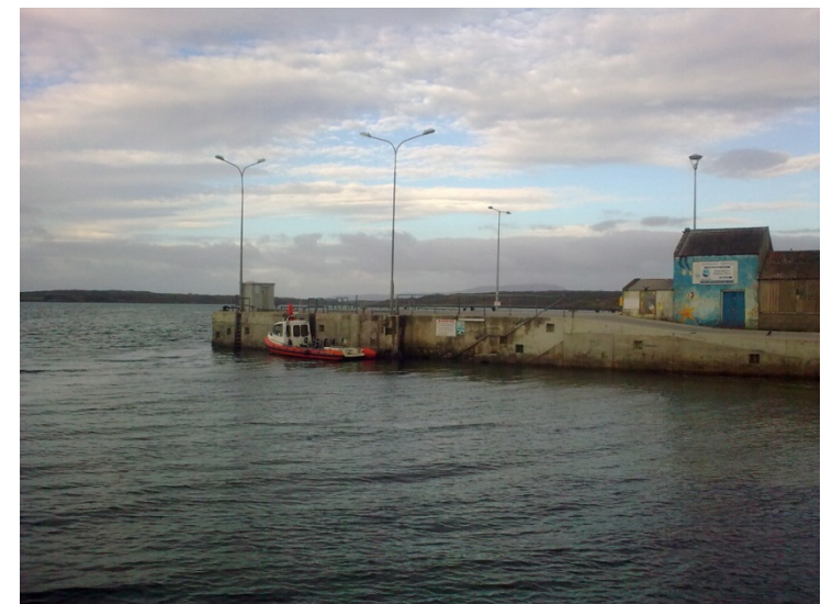
Figure 18: A Working Pier
